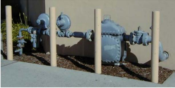
**Figure 7. Typical Diaphragm Meter Installation**
