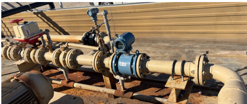
Figure 2. Examples of poor installations in produced water service
