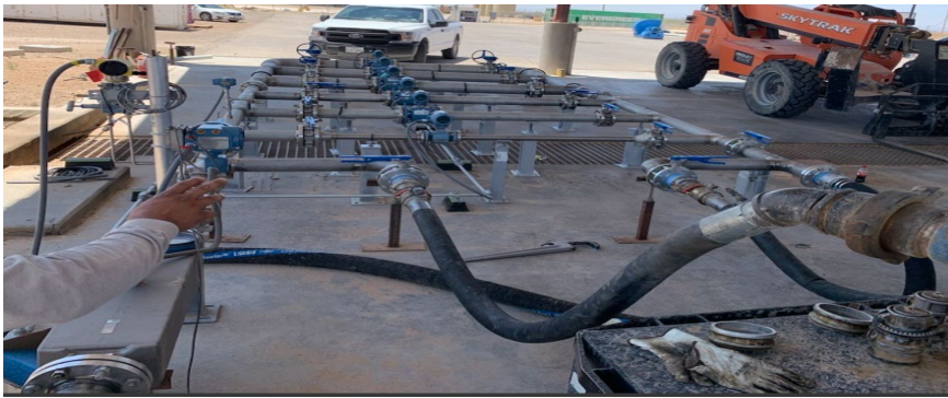
Figure 6. Internal proving loop with master meter
