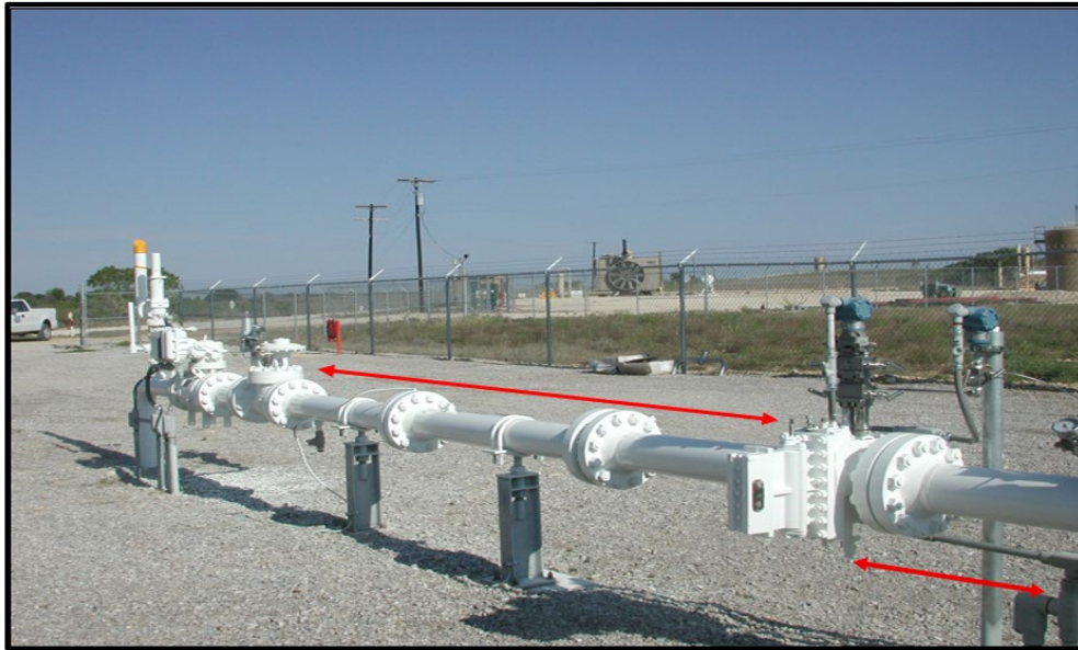
Figure 4. Upstream and downstream straight length verification.
