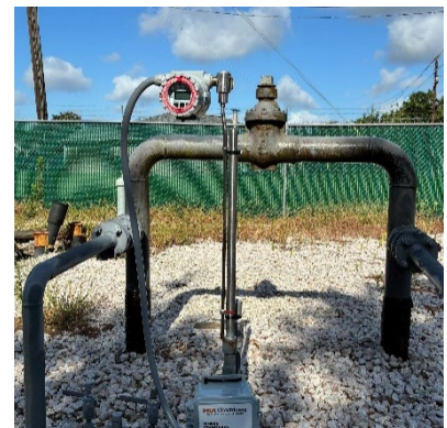
Figure 2: Watchtower Installed on 6B Kingtool, Buried
