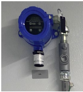
Figure 6 – Gas Detector
