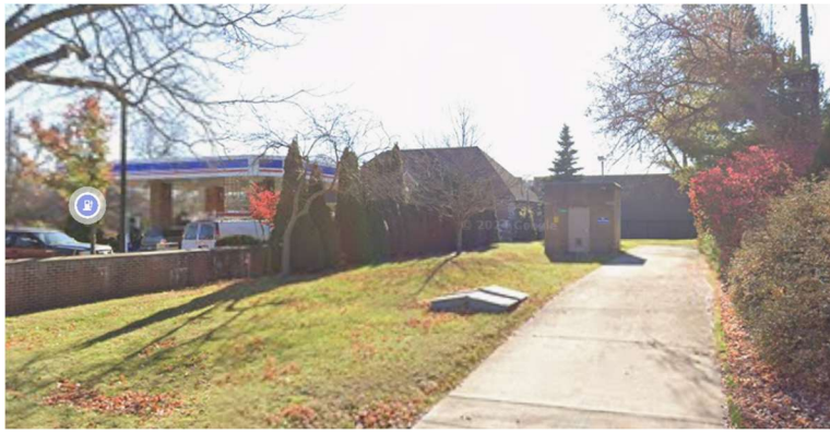
Figure 25: Regulation station before heater installation
