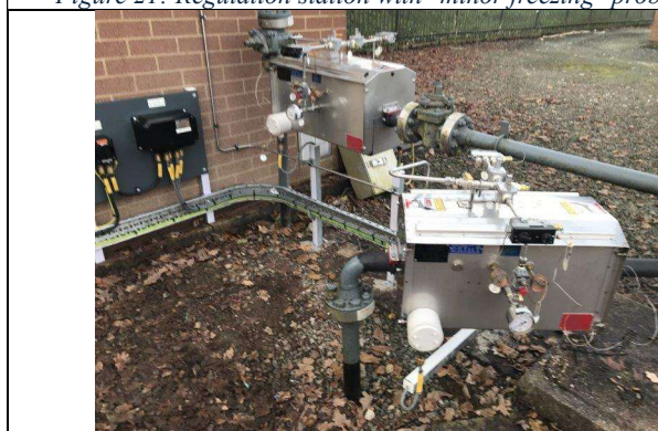
Figure 23: Catalytic Heaters (Twin-Paks) with 48,000 BTU input
