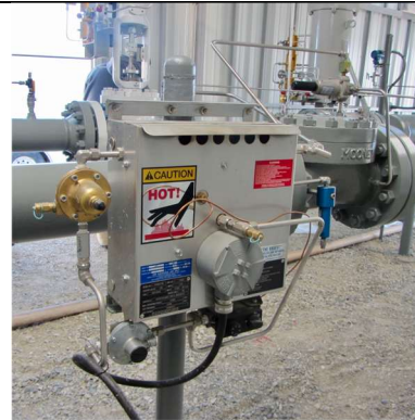
Figure 18: Single pilot heater
