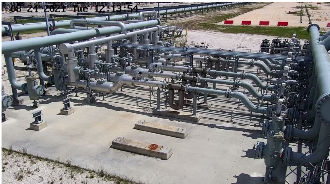
Figure 4 - Meters in Series with a Stationary Prover
