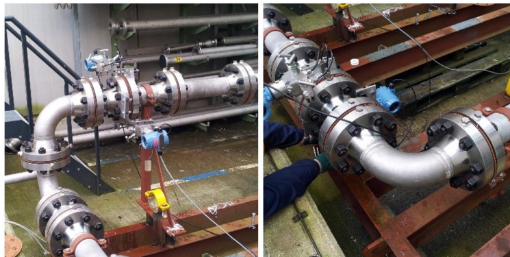
Figure 8 Double and single elbows near an orifice plate
