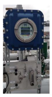
FIGURE (3)- HCD5000™ On-line Hydrocarbon Dewpoint Analyzer
