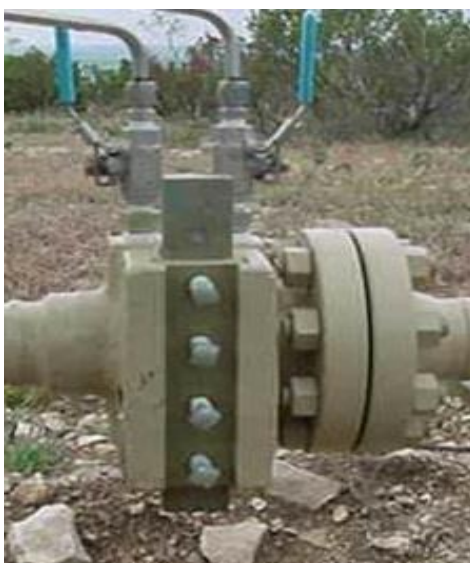
Figure 5. Single chamber fitting with flange tap valves
