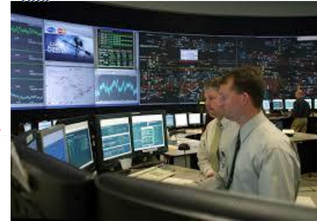
CONTROL CENTER 2 COMPUTERS AND HMI
