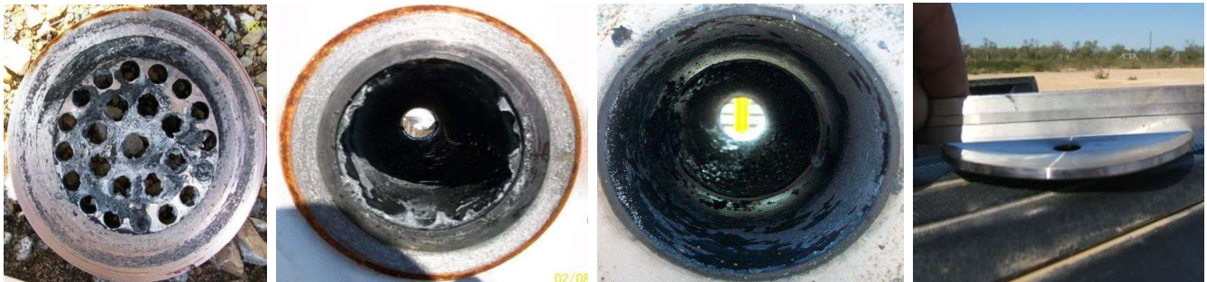
Fig. 3 Evidence of Liquid Flow through Orifice Meter
