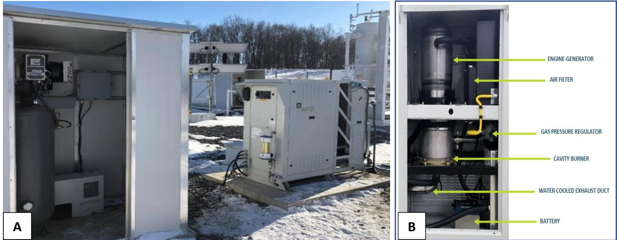
Figure 4. In field implementation of a Stirling engine driven air compressor system at a well site. (A) On left is cabinet housing compressor system with electrical power supplied by a cabinet (right) housing a Free Piston Stirling engine system connected to local natural gas. (B) shows the engine-generator internal housing.
