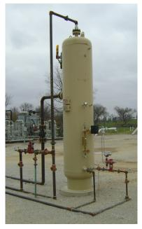
Figure 3. Example Gas-Liquid Separator System
