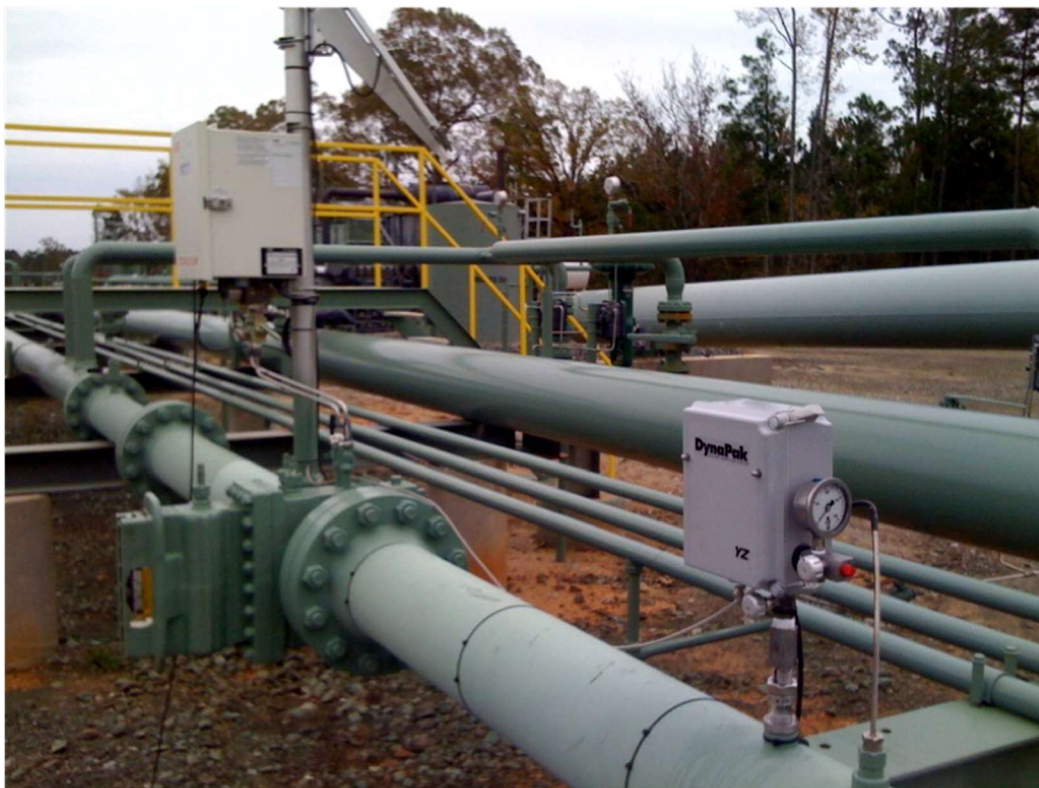
Figure 3; Direct Mounted Sampling System with EFM
