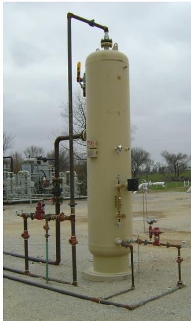
**Figure 3. Example Gas-Liquid Separator System**
