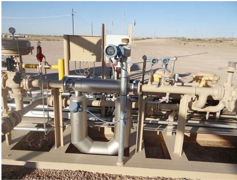
FIGURE 6: CORIOLIS METERS ARE COMMONLY USED
