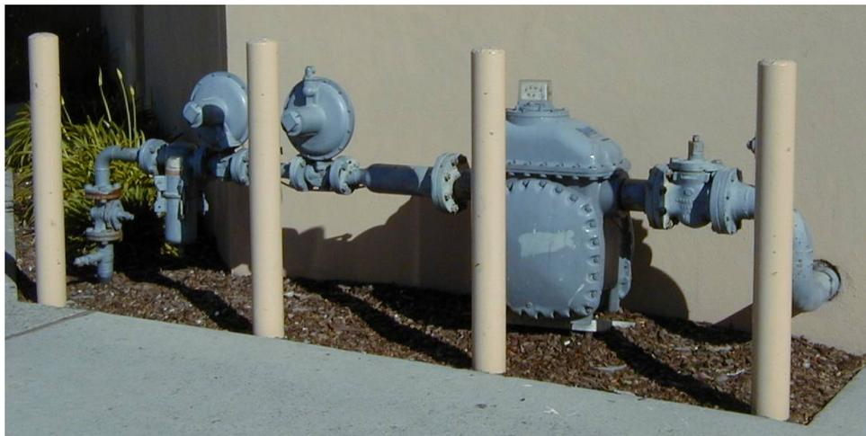
Figure 7. Typical Diaphragm Meter Installation
