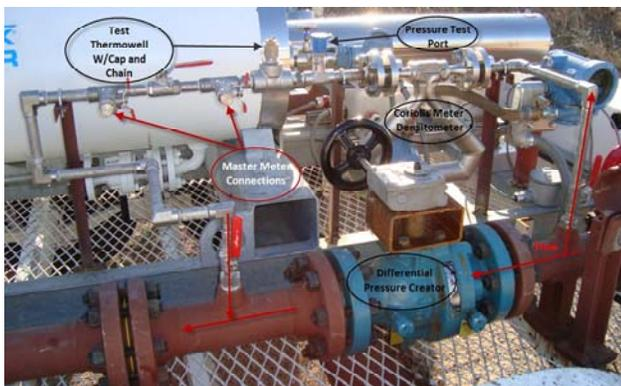
Figure 10 – Picture of a Flow through Denistometer Loop
