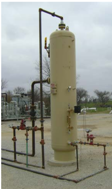
Figure 3. Example Gas-Liquid Separator System
