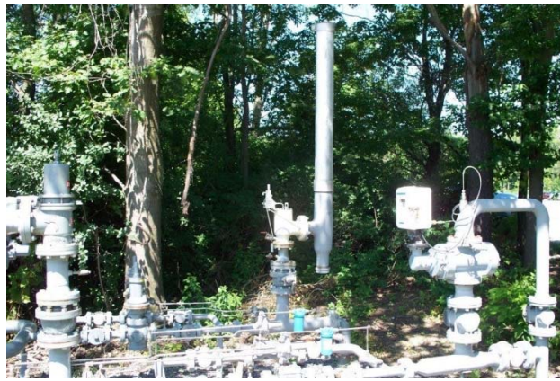
Figure 8. Typical PRV Installation
