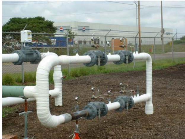
Figure 5. Regulator used as Relief
