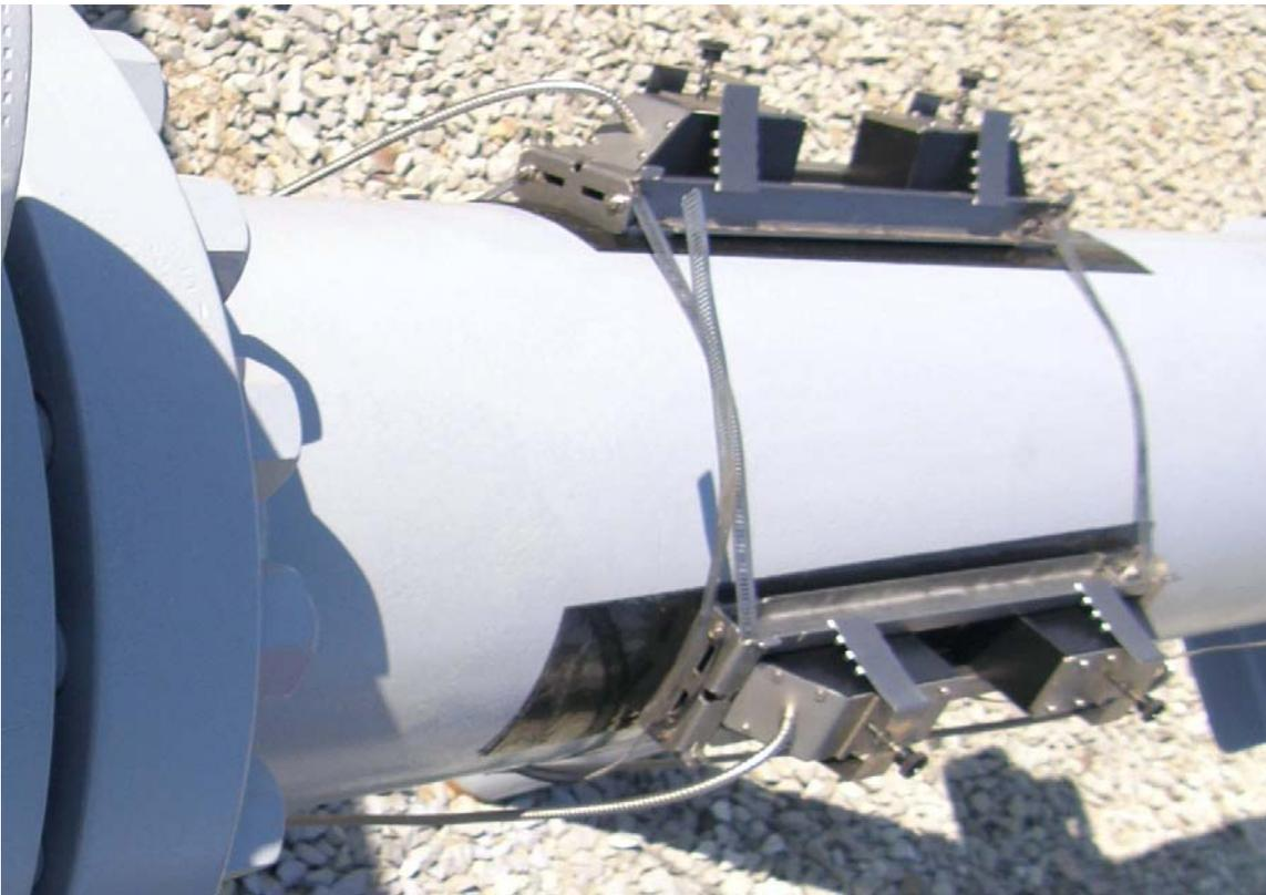
**Figure 5 – TRANSDUCERS MOUNTED ON PIPE IN REFLECT MODE**
