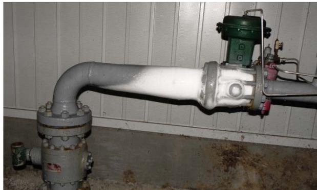
**Figure 13 - ICE IS CERTAIN LEAKAGE EVIDENCE**
