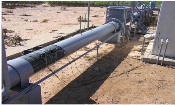
**Figure 9.-Clamp-on Compared to Orifice Meter**
