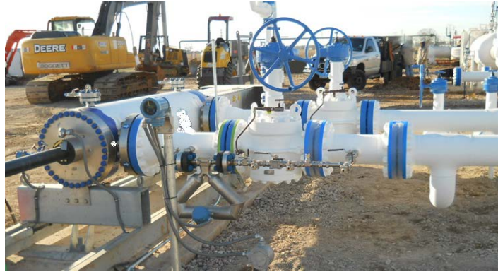
Figure 15 – Inferred Prover Installation
