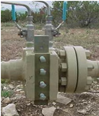
Single chamber fitting with flange tap valves
