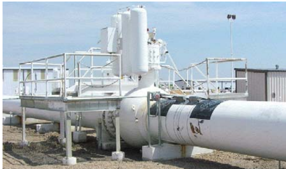
Figure VI. Permanent Segmentation Clamp-on
