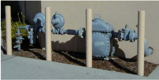
Figure 7. Typical Diaphragm Meter Installation
