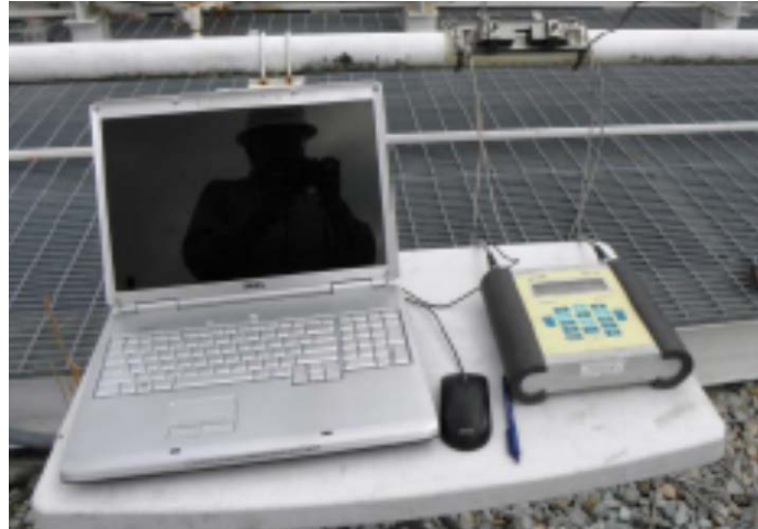
Figure XIII. – CLAMP ON DETECTION OF LEAK
