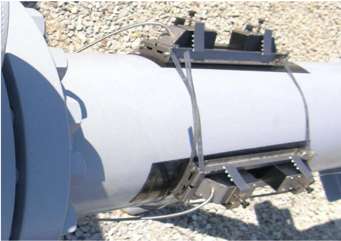
Figure V. – TRANSDUCERS MOUNTED ON PIPE IN REFLECT MODE
