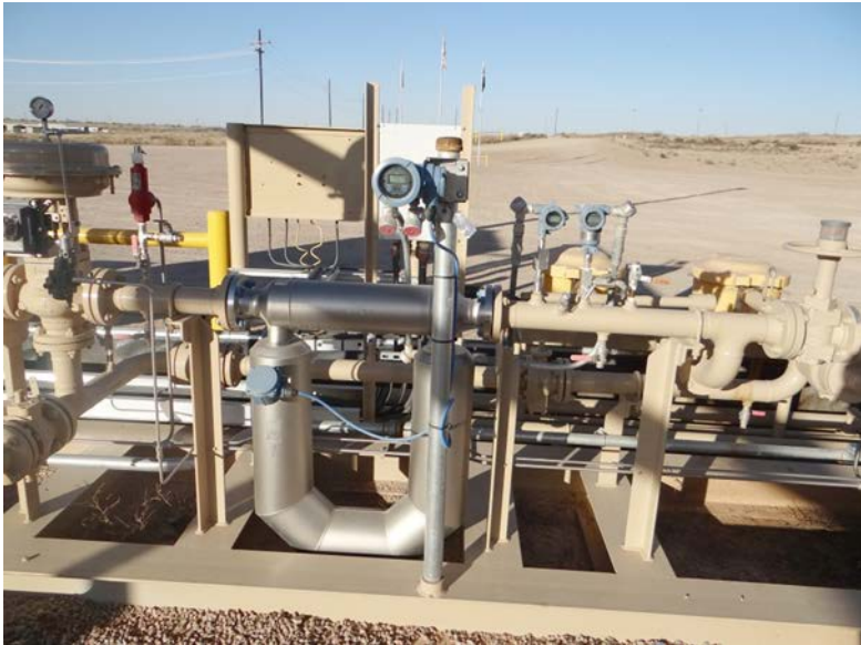
FIGURE 15. Coriolis Meters on LACT
