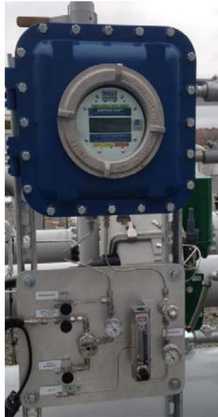
**FIGURE 3 - HCD5000™ On-line Hydrocarbon Dewpoint Analyzer**
