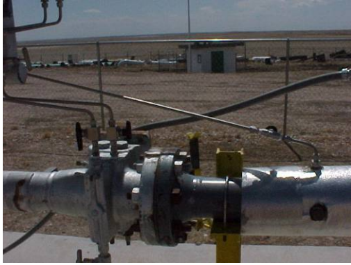
Fig 4. Orifice fitting with natural gas flow.
