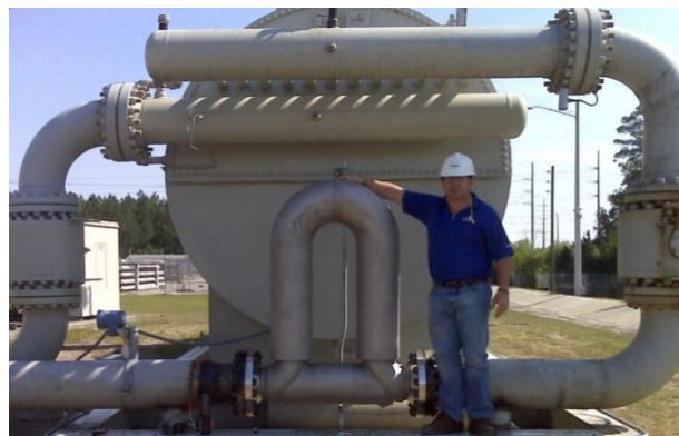
200mm (8") Coriolis meter installed in 250mm (12") line
