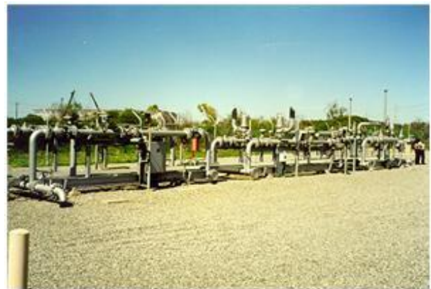
Western Australia: Previous installation using turbine meters for 50:1 turndown
