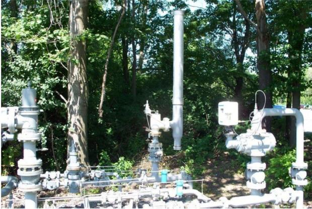
1. Inlet Line Loss - Riser Length: From the vessel or pipeline to the PRV - no more than 3% loss. Riser length must be examined to avoid harmonics.
