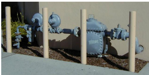
Figure 7. Typical Diaphragm Meter Installation
